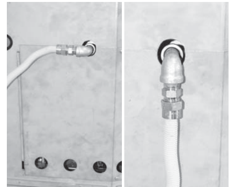
Flex connector redirected using two elbows.
