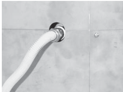
Flex connector redirected using one elbow.
