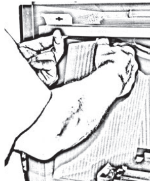
Rotate anchor up and insert panel
