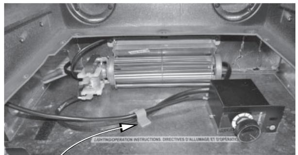
Clip thermoswitch wire and connector cable to sheet metal bottom using clip provided
