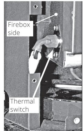
6. Use the U shaped self-adhesive cable retainer to hold the thermal switch wiring and connector cable to the bottom of the appliance and away from the fan inlet.
