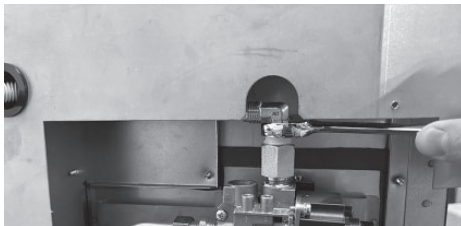
Flex connector redirected using one elbow.
