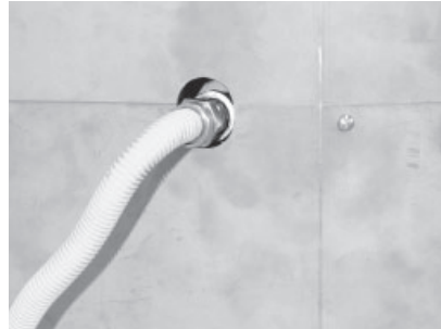
Flex connector redirected using one elbow.
