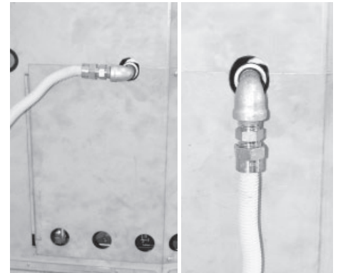
Flex connector redirected using two elbows.
