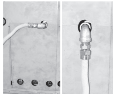
Flex connector redirected using two elbows.
