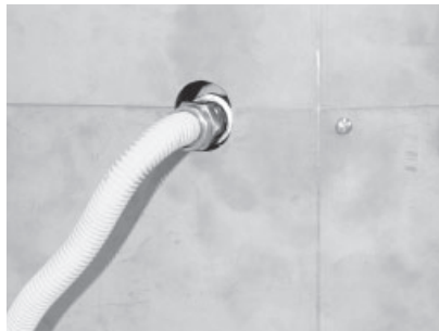
Flex connector redirected using one elbow.
