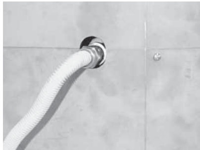
Flex connector redirected using one elbow.
