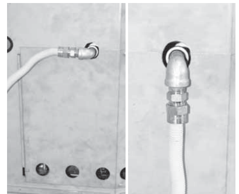
Flex connector redirected using two elbows.
