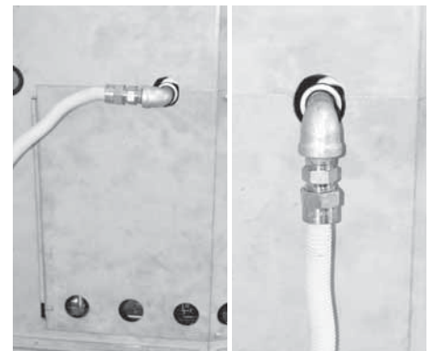
Flex connector redirected using two elbows.
