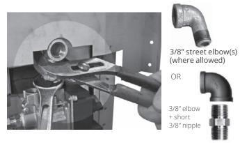
3. Re-install original supplied connector elbow.
