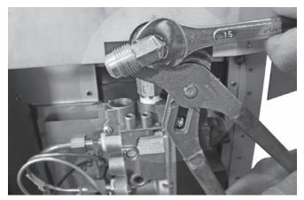
4. Install the flex connector to the alternate elbow.
