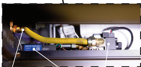
Gas Line Receiver Control Valve
