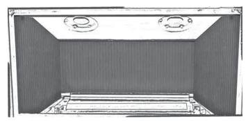
5. Tighten the side brick anchors on each side of the firebox.
