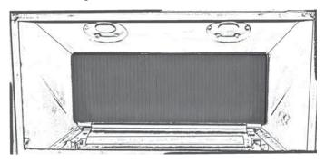
Rotate the anchor up and out of the way and slide the left hand side panel against the firebox side.
