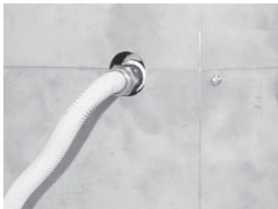
Flex connector redirected using one elbow.
