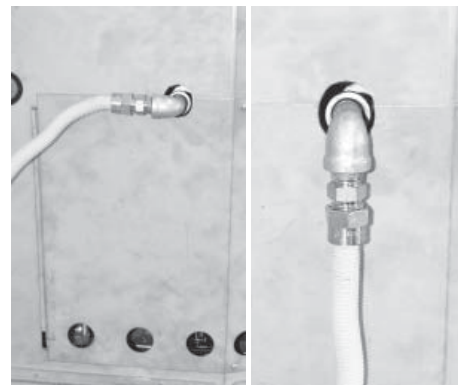
Flex connector redirected using two elbows.
